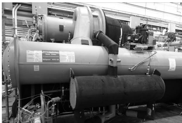
Image 3. One of two test chillers used to evaluate the performance and stability of R-514A.
